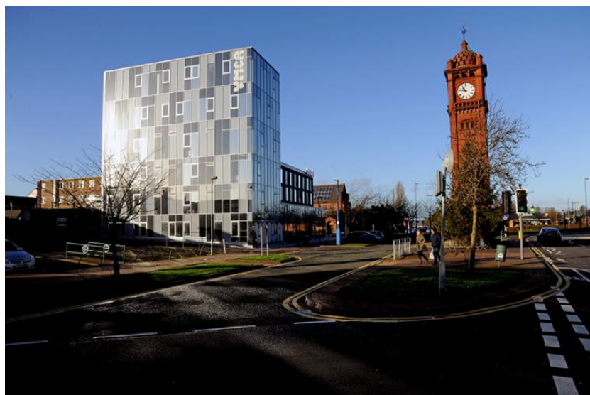
Figure 5. YMCA Western Gateway in West Bromwich
